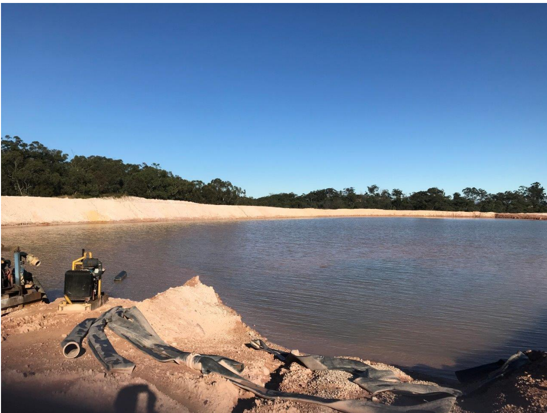
Plate 3 – Pit 14 Tailings Dam
