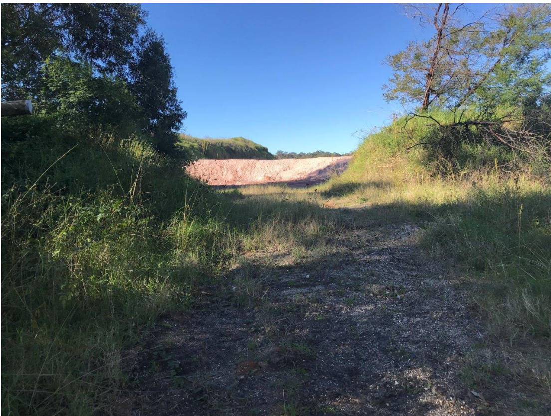
Plate 15 – Offset Bund installed post the 2017 IEA
