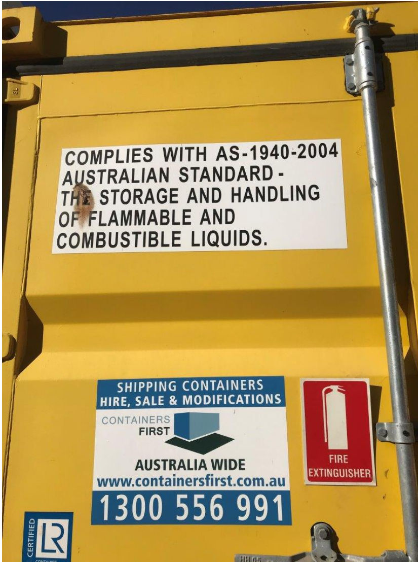
Plate 7 – Onsite Self Bunded Container for Machinery Lubricants
