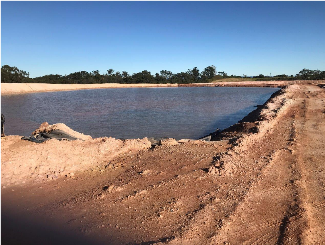
Plate 2 – Pit 14 Tailings Dam
