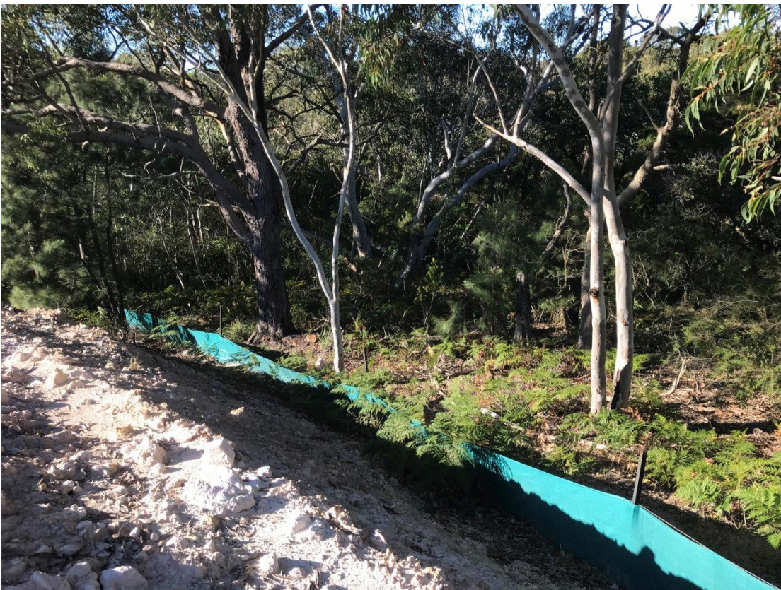
Plate 5 – Sediment Fencing adjacent to Pit 14 Tailings Dam
