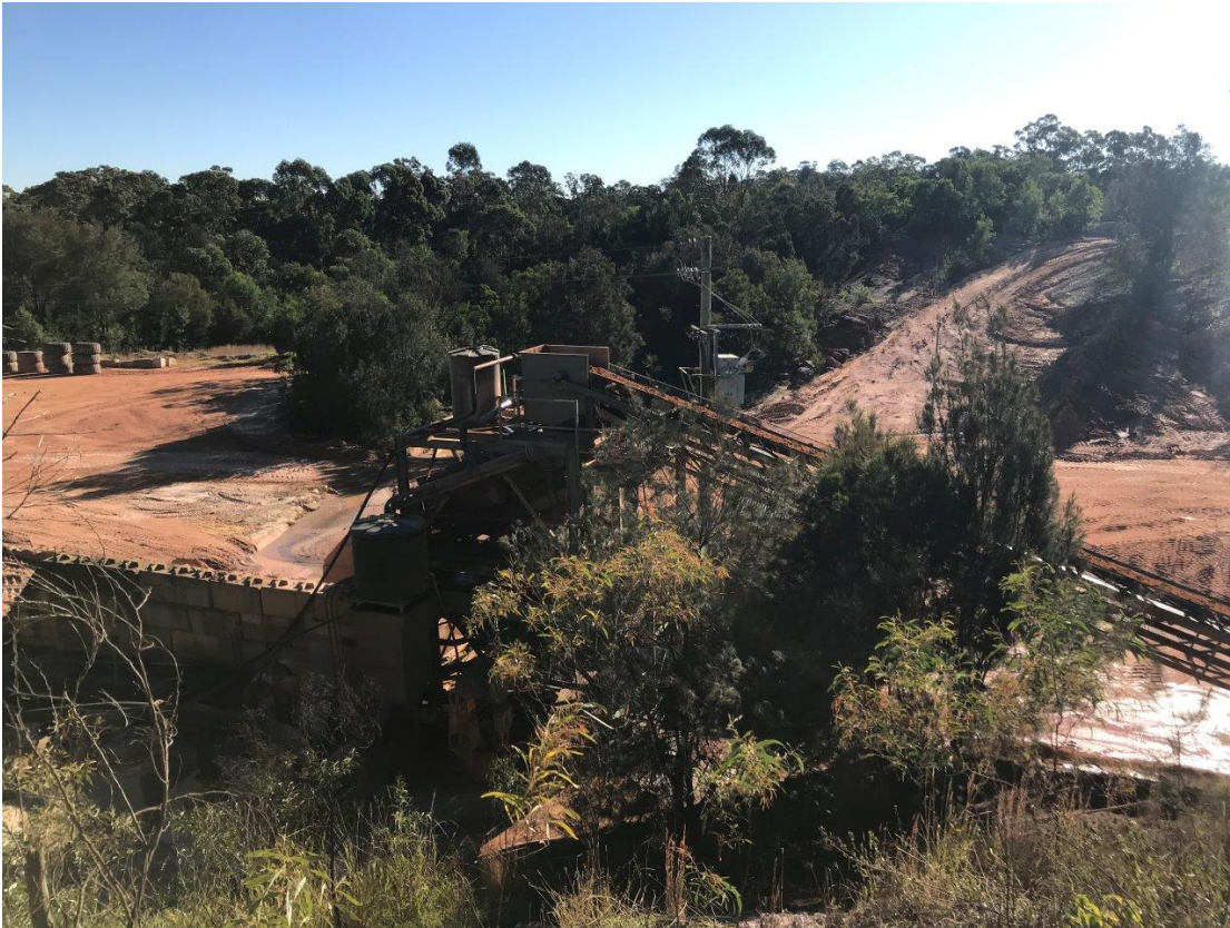
Plate 12 – Sand Processing Plant
