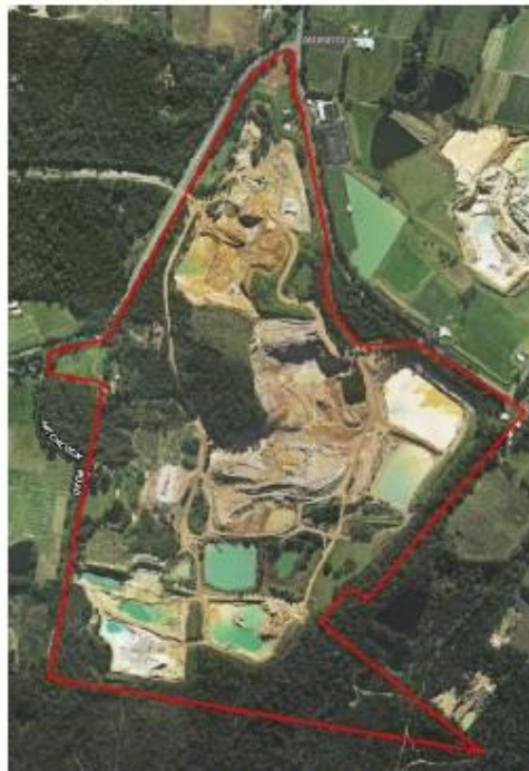
Figure 1. Hitchcock Road Sand Project Site Area
