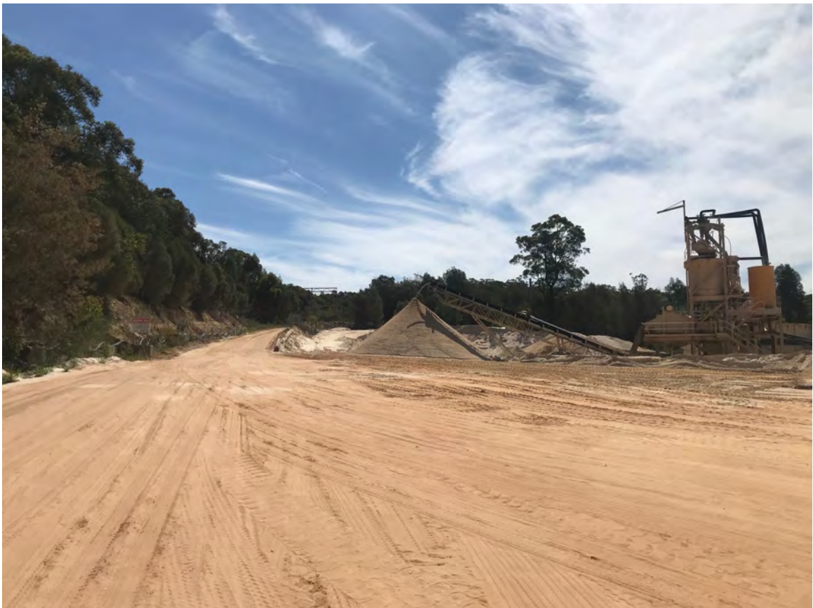
Figure 2 Existing Processing Plant Located on Lot 2 DP 748820
