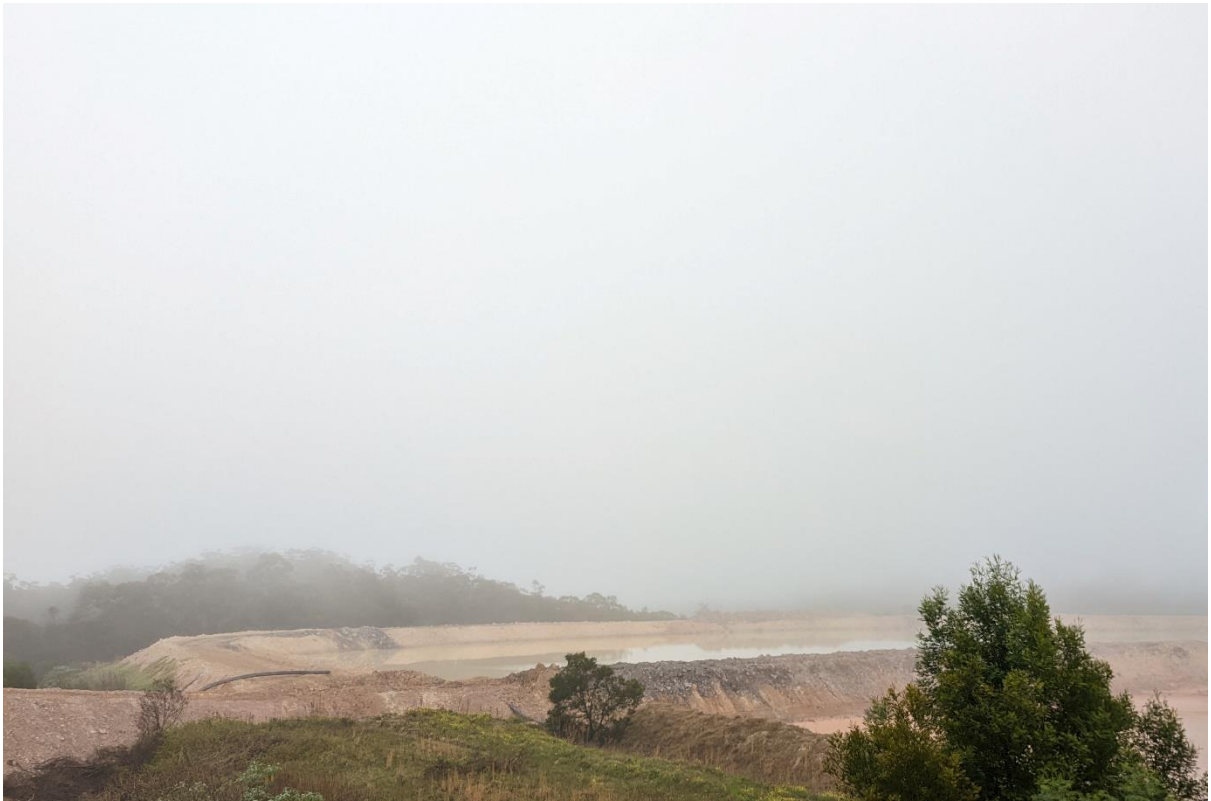
Tailings pond in use (13 + 14)
