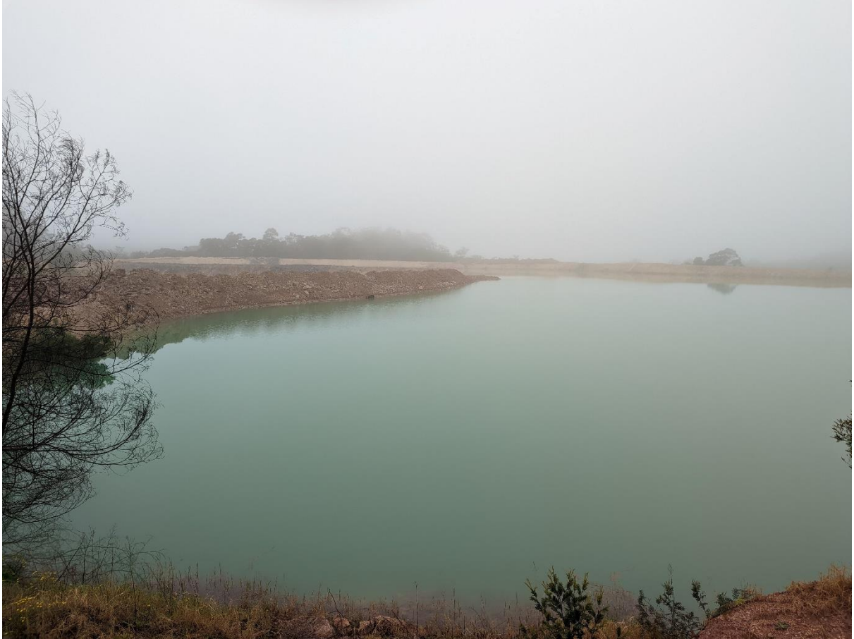
Tailings pond in use (13b)
