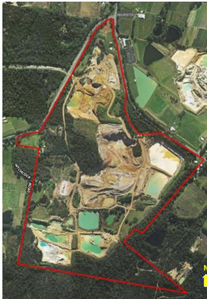
Figure 1. Hitchcock Road Sand Project Site Area
