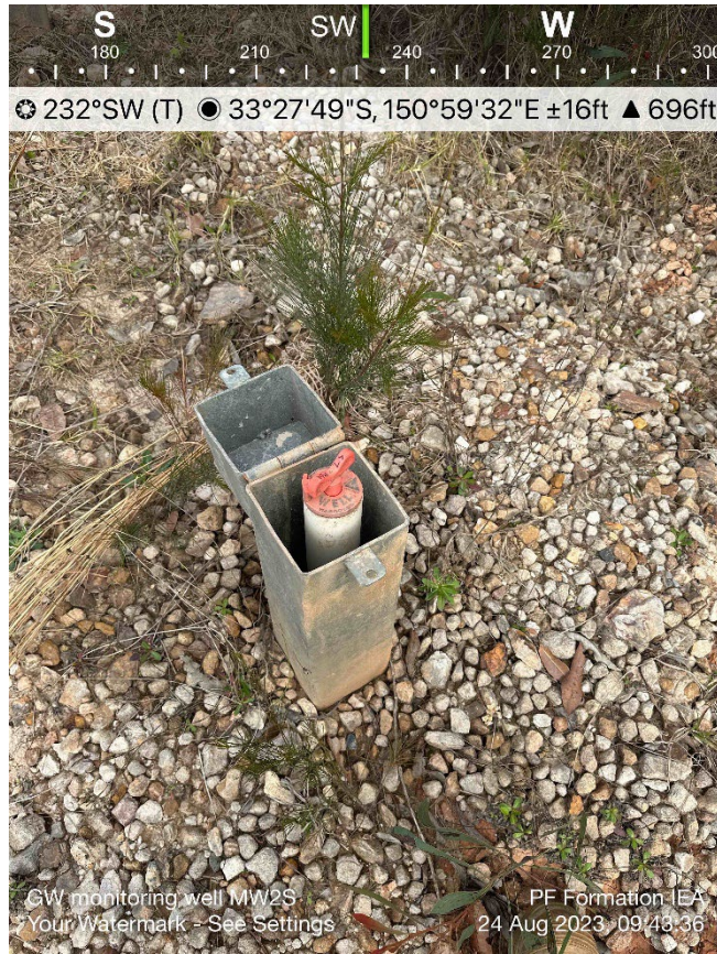
Plate 15 Groundwater Monitoring Well 2S
