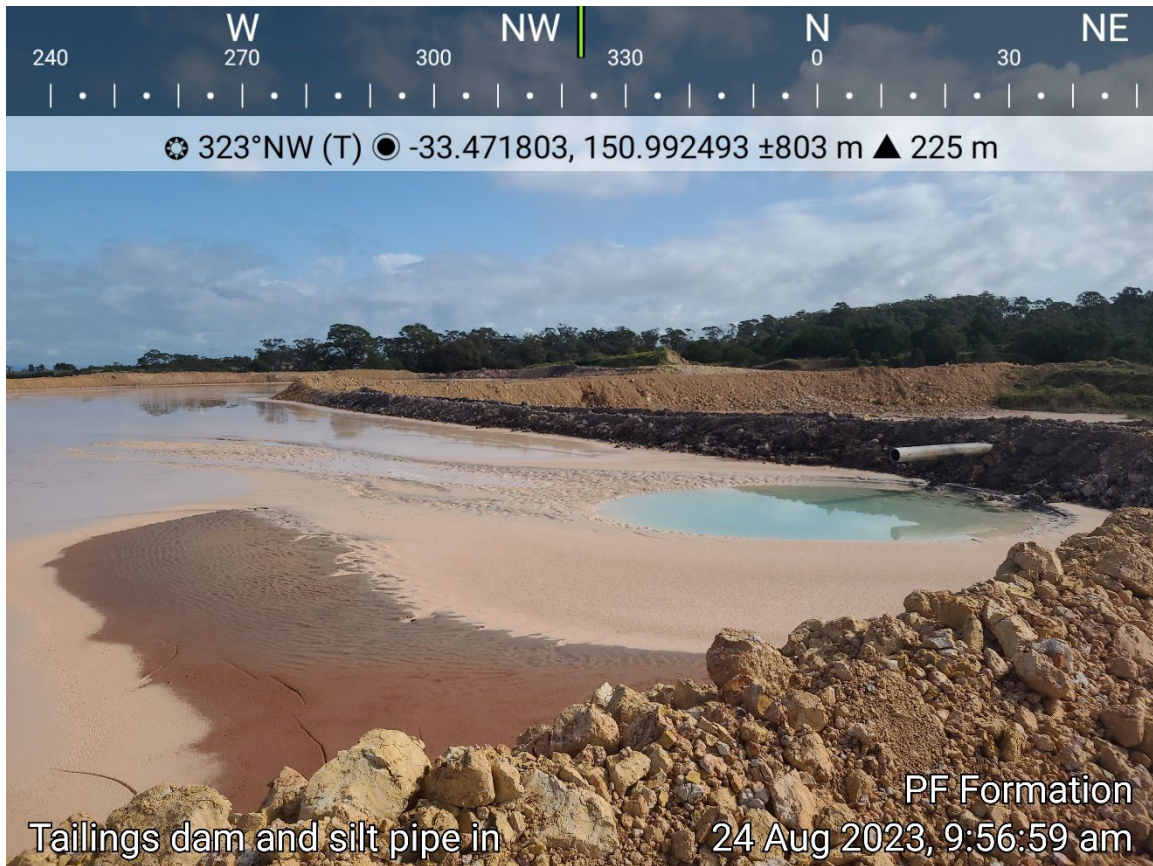
Plate 7 Tailings dam and silt inlet pipe
