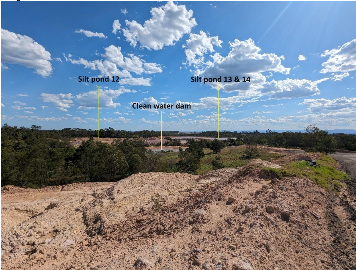
Tailings ponds in use 12, 13 and 14 with agricultural rehabilitation area and clean water dam in the foreground
