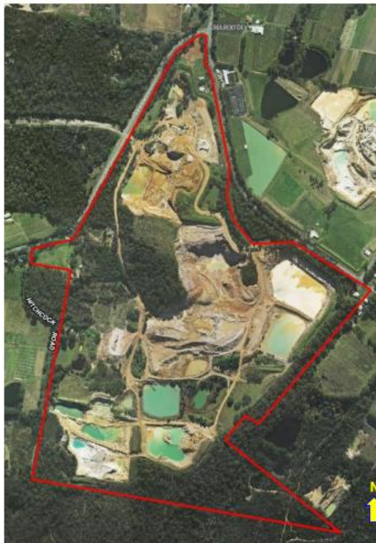
Figure 1. Hitchcock Road Sand Project Site Area
